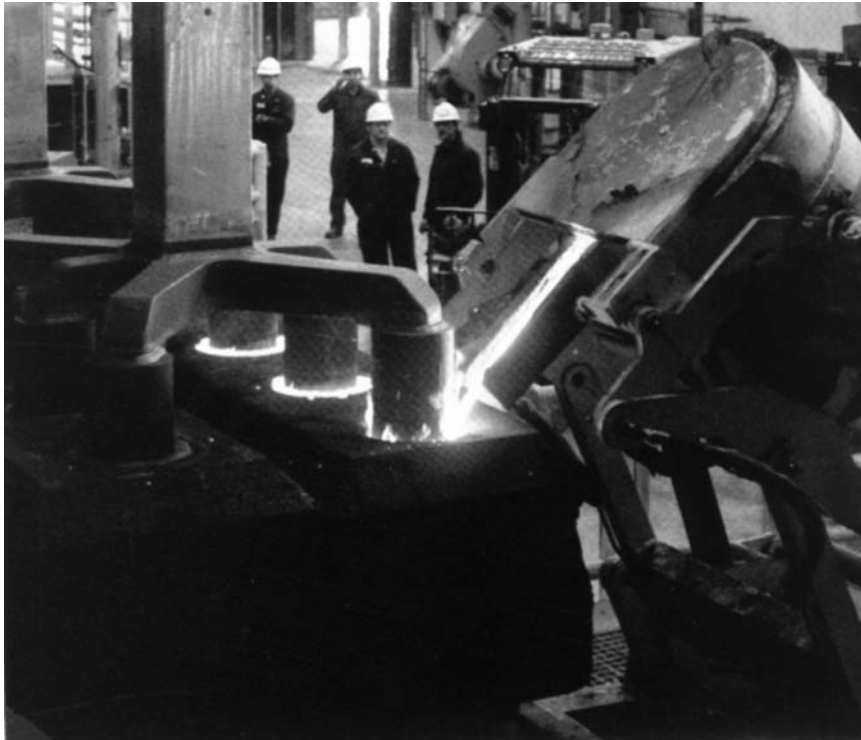
Figure 29 Fixing the rods in the anode blocks by pouring molten cast iron.
