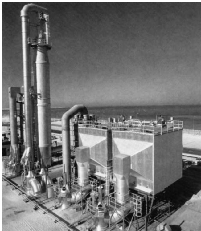
Figure 32 Fume treatment system for controlling anode-baking furnace emissions.
